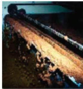
Skimmer boards remove sludge from the surface of the clarifier for transfer to the filter press.
