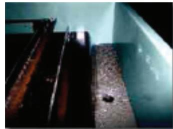
Clear treated water drains off from the clarifier for discharge to the sewer.
